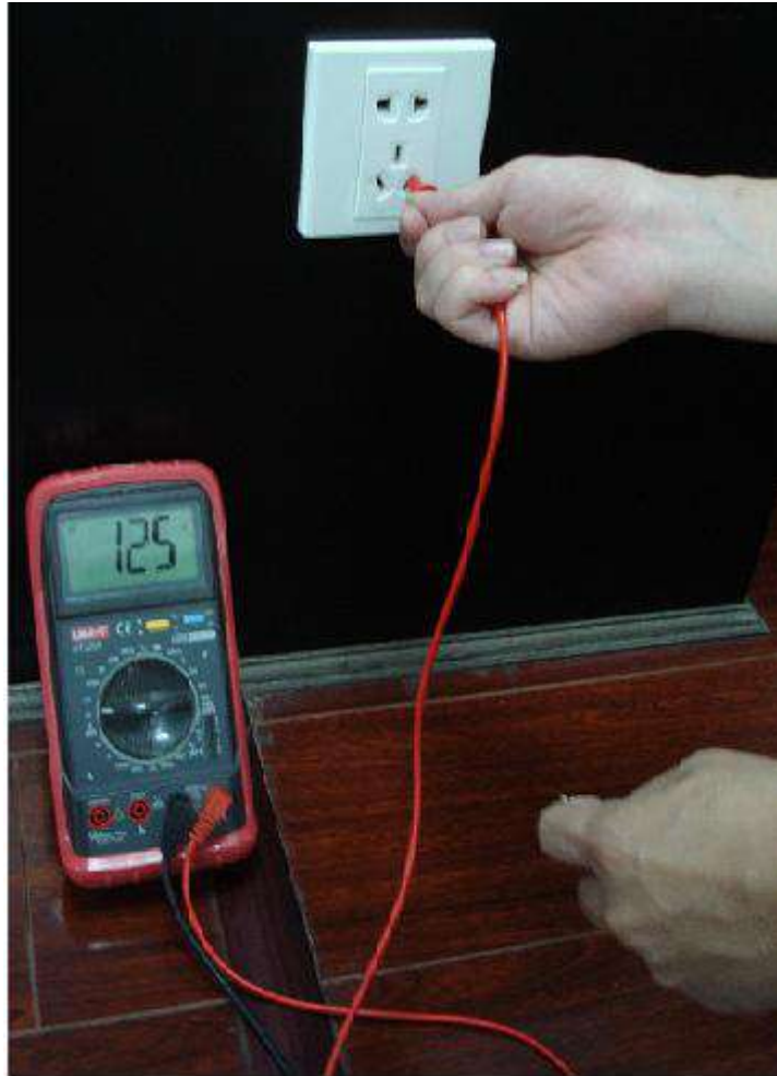
Appendix Figure 7-6 Check live cable connection
